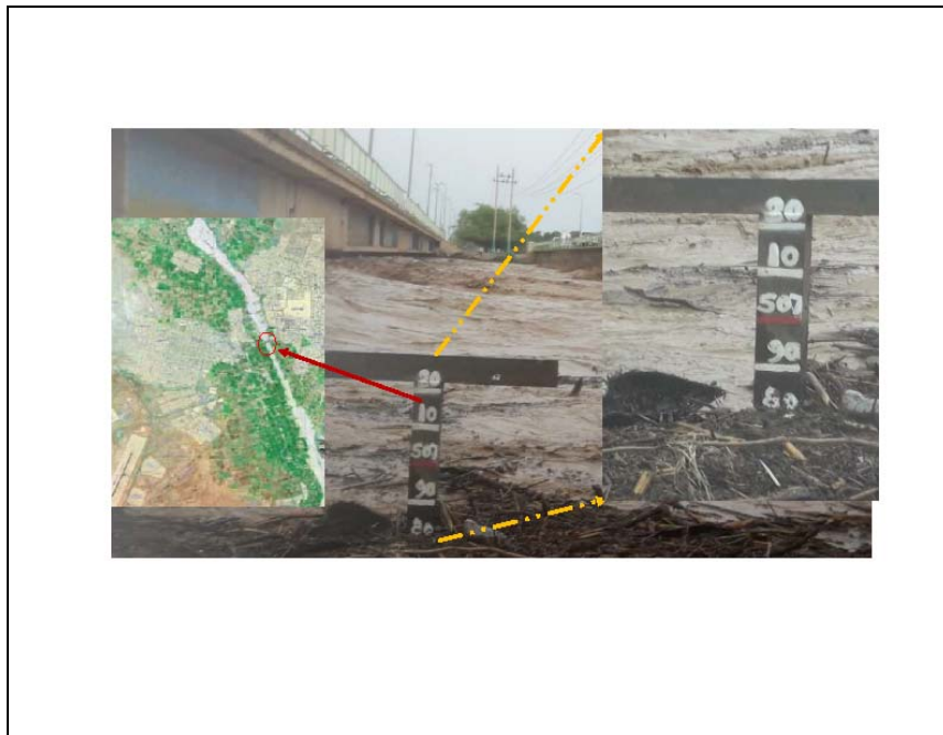
Figure 17: The alert level at Kassala Bridge gauging station.
